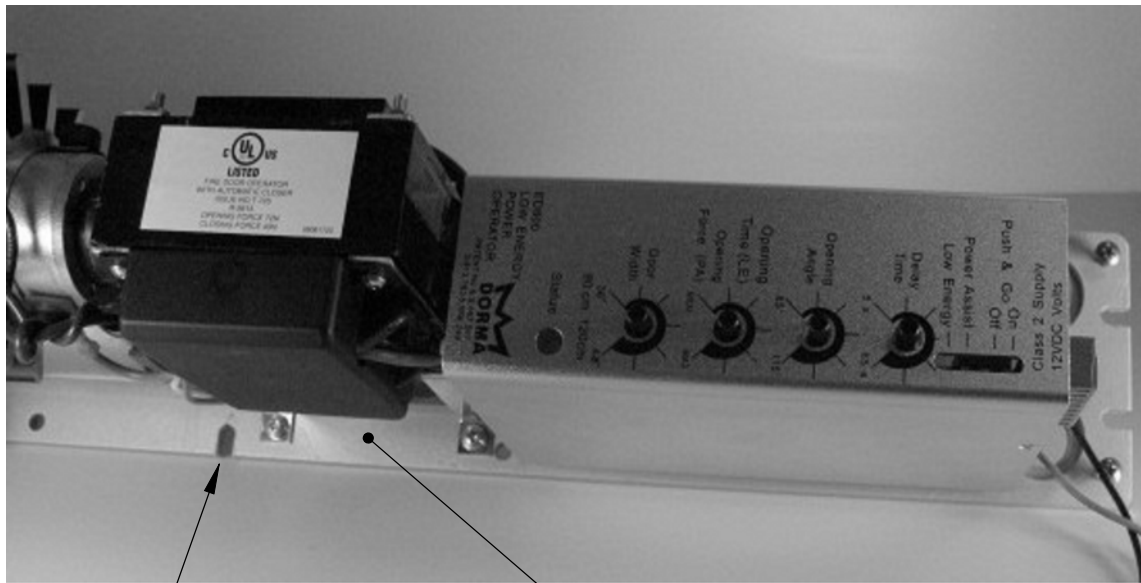
SLOT "A" — MOUNTING PLATE — SLOT "A" ← HINGE SIDE OF DOOR
