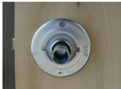
**Installed Spring Cage with Inside Spindle**
