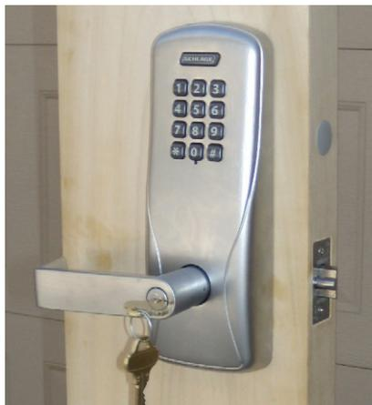
**Finished CO Lock Install Front View**
