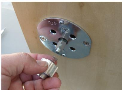
**Installing Spindle Cam**
