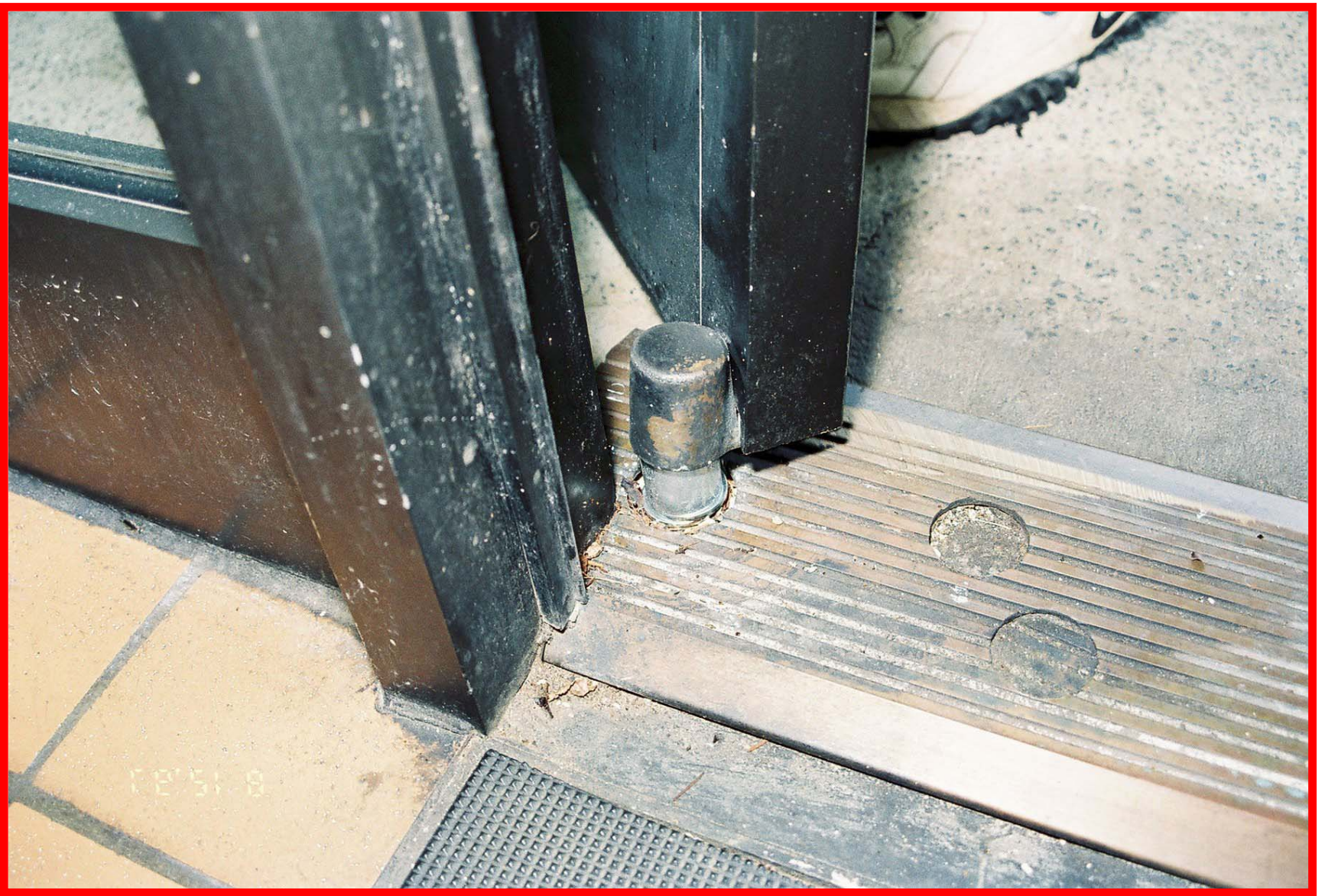
Lifting Door Off of Off-set Pivot!
